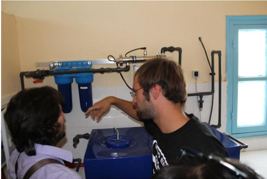
After the workshop, most of the participants visited the membrane distillation system in Jdairia-El Bibène, which has been installed within the MEDIRAS project. An Oryx unit of 150 liters per day has been installed in the roof the local health centre. The fresh water tank has been installed in the kitchen of the hospital together with a remineralisation system and a disinfection system which re-circulates the water through the UV lamp.
